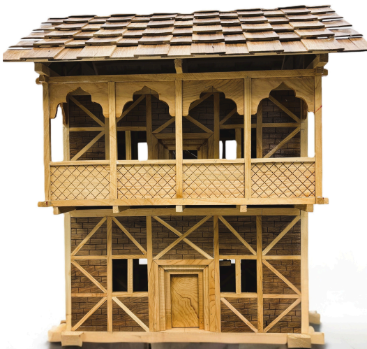
3D model of a traditional Dhajji-Dewari building system.
