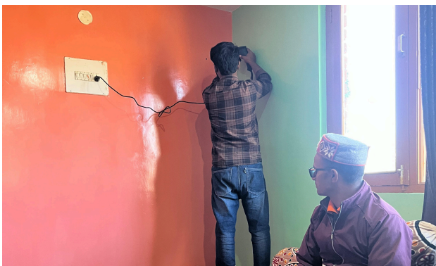
Installation of sensors in a traditional RC building.
