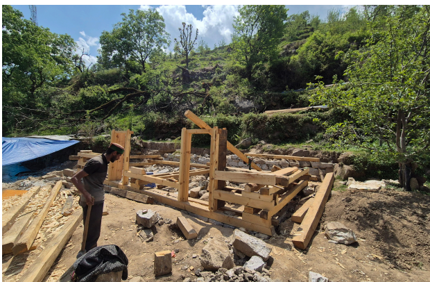
Local artisan engaged in traditional construction practices on site.
