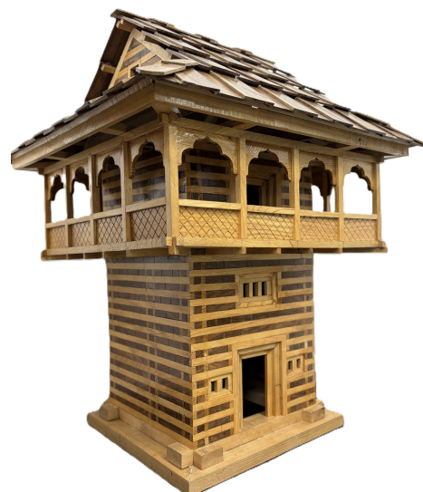
3D model of a traditional Kath-Kunni building system.
