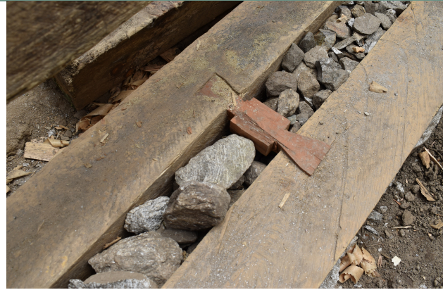
Close-up of timber bands and stone joints forming the seismic-strengthening core of Kath-Kunni construction.
