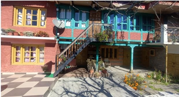
RC structure where sensors have been installed to monitor climate-responsive parameters, enabling comparison with modern buildings.
