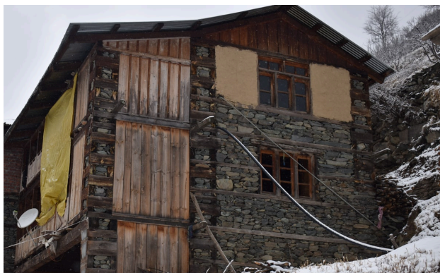
Traditional Thathara building
