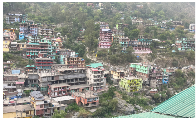
Modern RCC interventions within traditional settlements.
