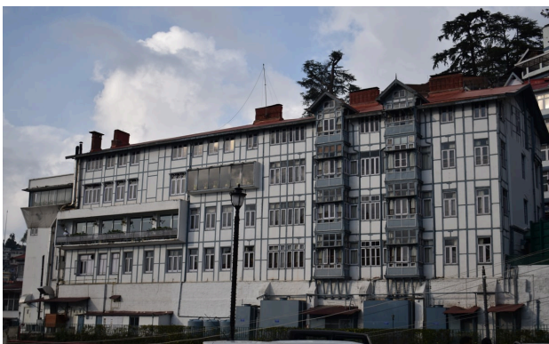
Traditional Dhajji Dewari Building
