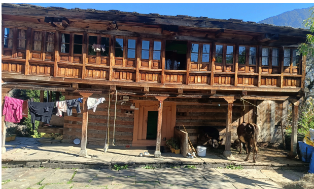
Kath-Kunni building fitted with sensors to track climate performance and compare with modern buildings
